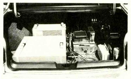
The Buicks' trunk was filled with electronic gear including two Pentium PCs. In the future, the technology would be made much smaller and integrated into the car's on-board computer.
