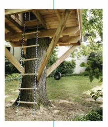
tree-hugger engineering -> My daughter Eliot (left) performed a supervisory role during the construction. When constructing the roof, I flashed the gap between the cedar shakes and the tree using a truck tire's inner tube, secured with a bungee cord (above, left). A rustic ladder made of 34-inch nylon rope and 134-inch dowels provides access—or, when hoisted up, thwarts invaders from terra firma (above, right).
