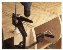
3 SCREW THE SHELVES • I used an "L"-shaped piece of plywood to keep my shelves square to the bottom as I fastened the shelves. Clamp it to the shelf and back as shown then screw the shelves in place.
