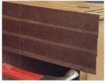
5ATTACH YOUR SIDING • After the first piece is in place, use a 15/8" wide spacer block to mark a pencil line at each shelf location to give you the location of the next piece of siding. Apply adhesive to the edge of each shelf where the strip will be nailed. Use only one nail at each shelf and two nails at the stern and stem. Locate the nails so that they are covered by the next strip.
