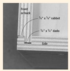
A simple and very common drawer joint in commercial furniture is the tongue-and-rabbet (or dado-and-rabbet) joint. It's made by simply running a dado in the drawer sides and then rabbets on the drawer fronts and backs. Both operations are best made with a router in a table.
