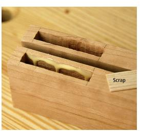
A thick bead of glue at the top of the mortise wall makes the joint strong without squeezing out a lot of glue. Use a small piece of scrap to paint the mortise wall before inserting the tenon.
