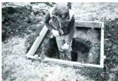
The hole for the pad was slightly deeper than 3ft at the deepest point. Note the terracing of the hole.
