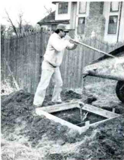
The concrete is poured, leveled and allowed to set for at least two days.
