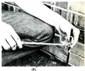
Fig. 10 A good ground, having highcurrent capacity, is necessary for protection of the CB equipment. Drive a 6-foot copper stake into the ground at a point near the antenna mast. (photo A). Firmly bond the ground wire to the mast and run it (as straight as possible) to the stake (B), avoiding metal gutters wherever possible.
