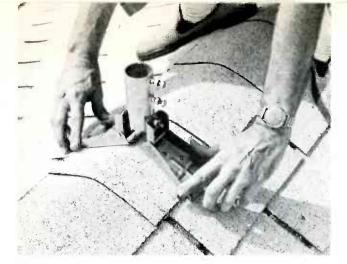
Fig. 1 Locate a spot at the ridge where two rafters meet, so all the screws can bite into solid wood. This is a saddle mount.
