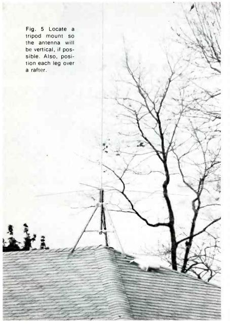
so all the lag screws bite into solid wood. This is most likely at a spot where a pair of rafters join the ridge. You can "probe" for solid wood by hammering a slim screwdriver bit or a nail-set punch into the roof till you find solid rafter. (Be sure it's not just the plywood roof sheathing.) Holes made this way and not used are easily sealed.
