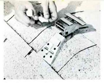
Fig. 2 On the bottom of the saddle mount, cover the screw holes with self-sticking tape, which prevents water from entering.
