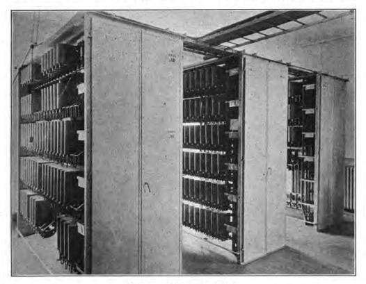
FIG. 98.-Selectors installed.
