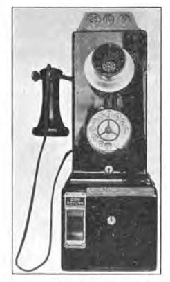
FIG. 182.—Three-slot coin box telephone.
