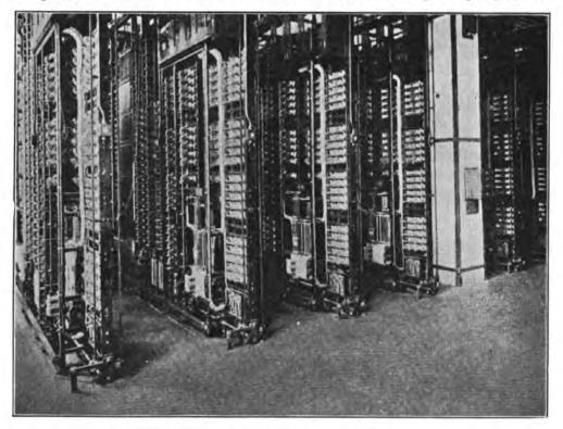
FIG. 216.-General view of panel type switch installation.
