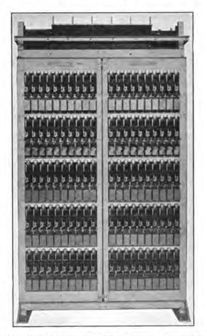
FIG. 88.-One-hundred-line switchboard, rotary lineswitches (front).
