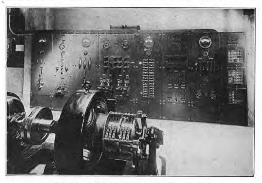
FIG. 280.—Power switchboard and charging machine.
