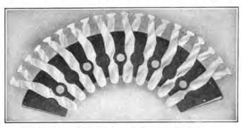
FIG. 56.—Detail of connector-switch bank.
