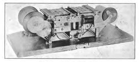
FIG. 302.-Traffic recording machine.
