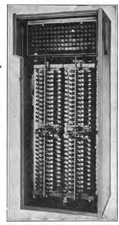
FIG. 175.—Lineswitch unit with meters at top.
