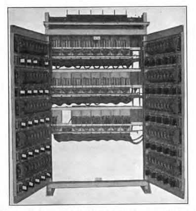
FIG. 89.-One-hundred-line switchboard, rotary lineswitches (front open).
