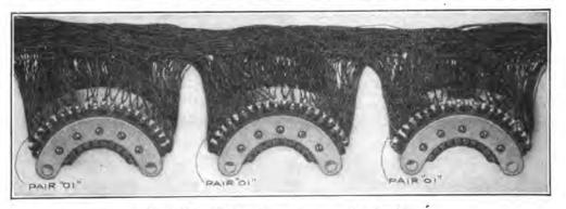
FIG. 57.-Wiring of connector-switch banks.
