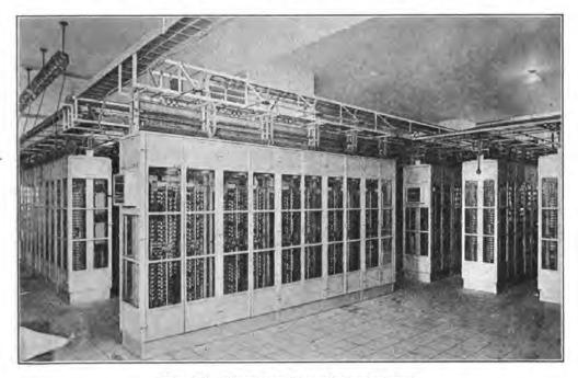
FIG. 95.—Secondary lineswitches installed.
