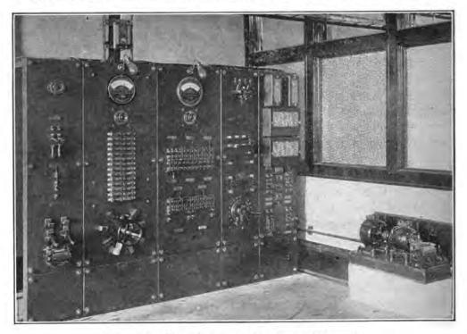
FIG. 279.—Typical power and battery switchboard.
