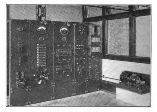
FIG. 239.—Typical power and battery switchboard.
