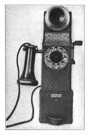
FIG. 83.-A combination telephone and coin collector for both local and toll-line service.
