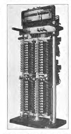
FIG. 37.—Keith line switch unit carrying roo-line switches.
