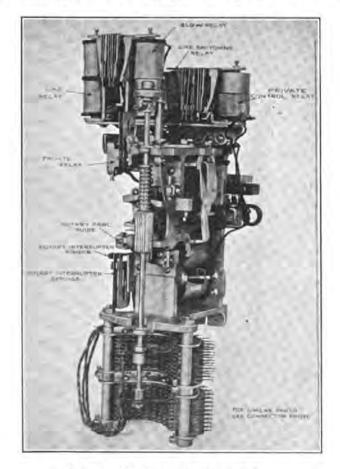
FIG. 54.-Two-wire selector switch.
