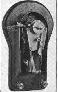
impulses followed by a rest, succeeded by another set of ten, indefinitely. One button operates the switch through zero loop resistance with 2 m.f. across the line, the other through 1200 ohms without capacity. A release button opens the line to release the switch. Another button cuts 130 ohms in series with the motor armature, slowing it down to five impulses per second.
