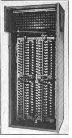
FIG. 78.—Line switch unit with meters at top.
