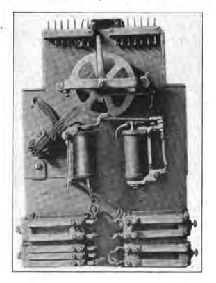
FIG. 91.-Finder switch with magnets and relays.
